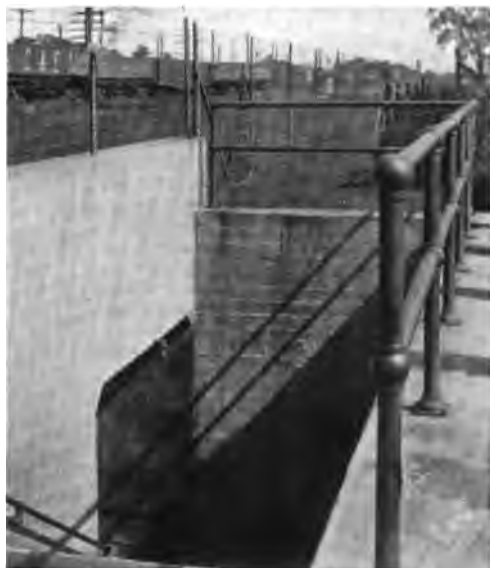
Fig. 1. Subway at Plant Entrance.*
